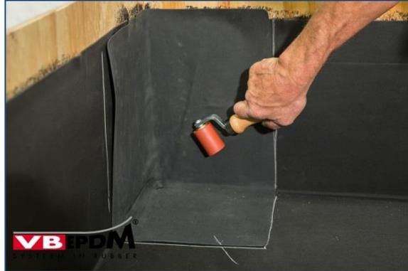
60. Rolling sealing sleeve with silicone roller.
