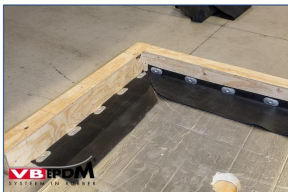
36. Reinforced EPDM strip as perimeter fastening.
