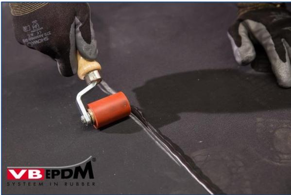
166. Rolling repair piece with silicone roller.
