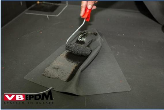
57. Gluing in sealing sleeve.
