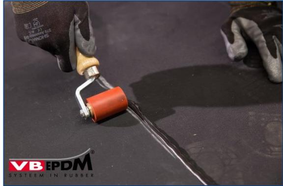
25. Rolling adhesive/sealant seam with silicone roller.
