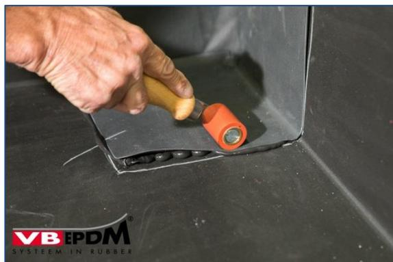
62. Roll the sealed part with silicone roller.
