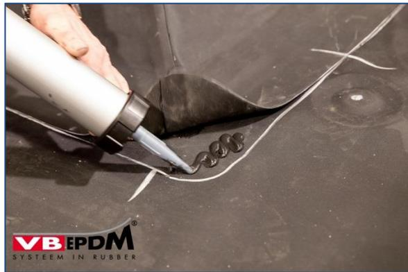
137. Bottom side of sealing sleeve sealed with VB-9510.
