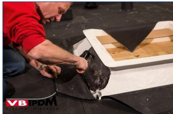
118. Gluing in dome upstand with adhesive-free zone.
