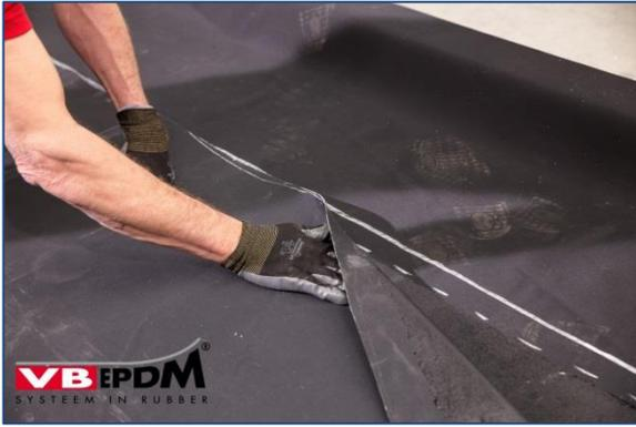
22. Folding VB-EPDM seam joint shut.
