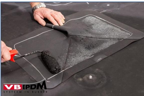
71. Gluing in prefab outer corner piece.
