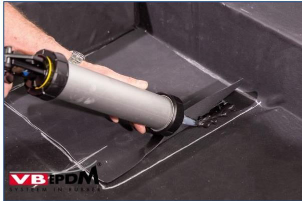
145. Sealing flashing with VB-9510.
