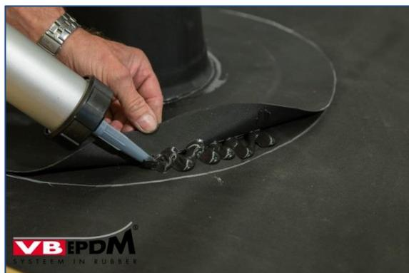
99. Sealing with VB-9510 in the roof plane.
