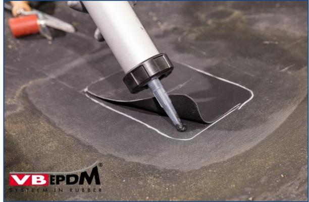
165. Sealing repair piece with VB-9510.
