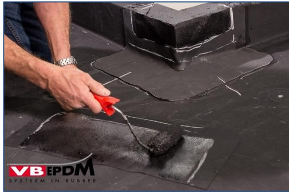
81. Gluing in corner sealing sleeve and substrate.
