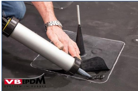
108. Sealing the sealing sleeve with VB-9510.
