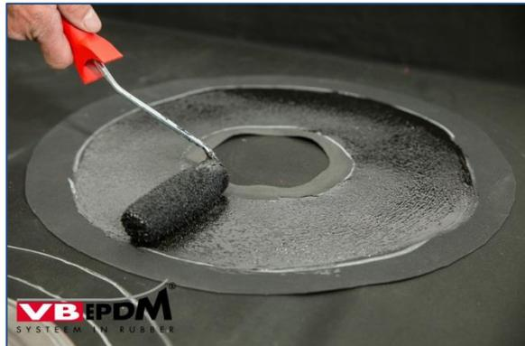
89. Gluing in sealing sleeve.
