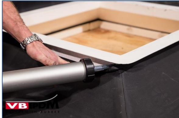
135. Top side of sealing sleeve sealed with VB-9510.
