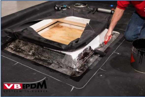
132. Gluing in sealing sleeve + dome upstand.
