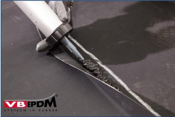
24. VB-9510 rubber sealant applied zigzagged.
