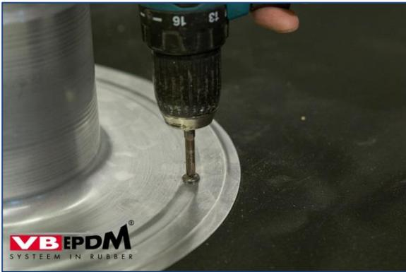
84. Mechanically fixing lead-through.
