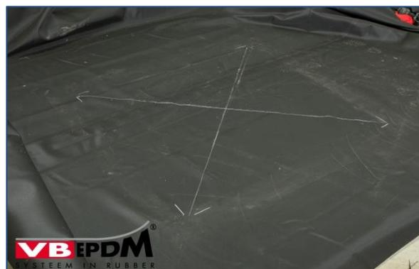
112. Cutting into membrane (**Note protection against falling!**).
