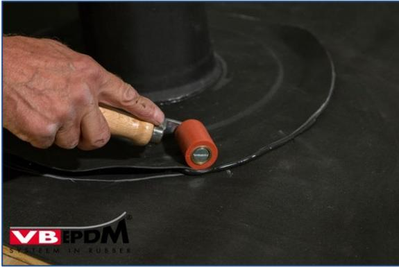
100. Rolling seal seam with silicone roller.
