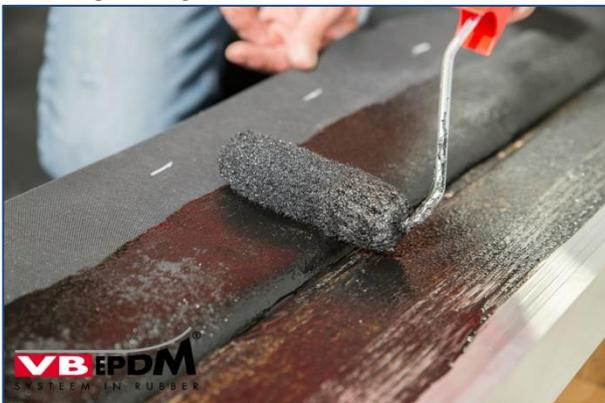
149. Gluing in roof trim + membrane.
