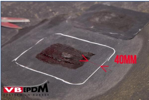
164. Gluing in place of the repairs and repair piece.
